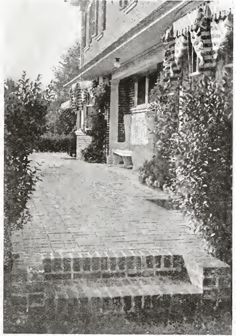
Terrace—Residence of Frederick Stout, Esq. Ardmore, Pa. H. W. Sellers, Architect.
